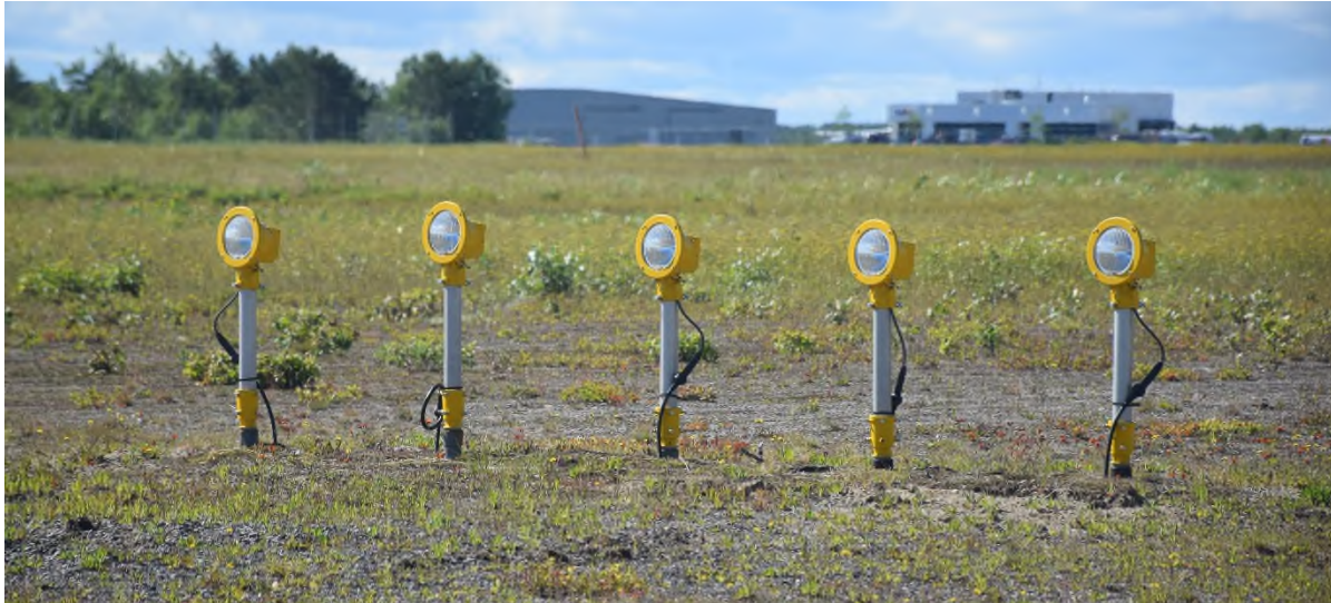
Figure 478 - Short Simplified Approach Lighting with Runway Alignment Indicator Lights (SSALR) Row of White Lights
