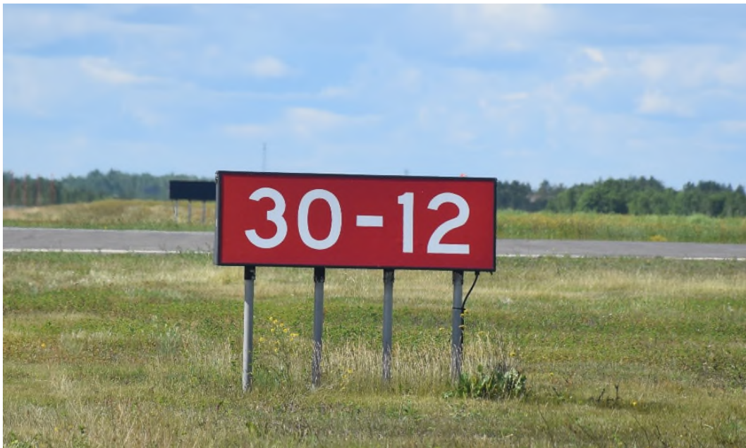
Figure 12 - Runway-Runway Intersection Mandatory Instruction Sign
