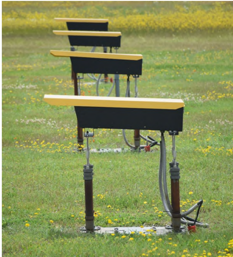
Figure 434 - Precision Approach Path Indicator (PAPI) Side View
