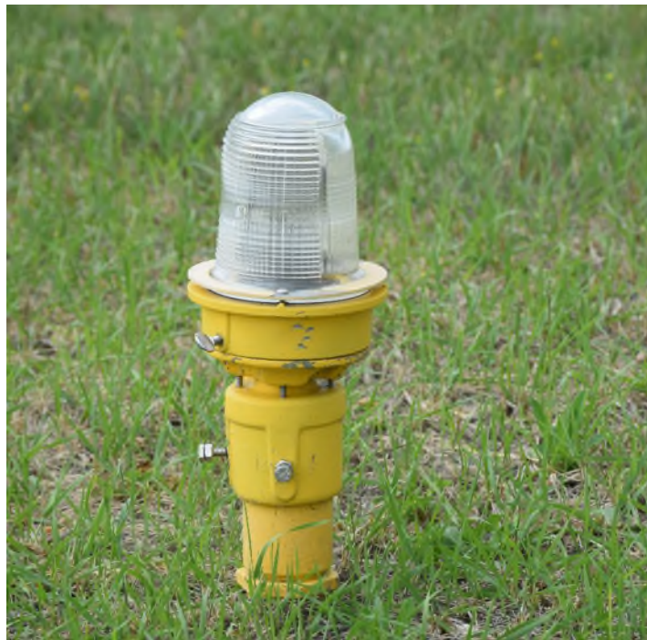
Figure 23 – Runway Edge Light located on Runway 12-30
