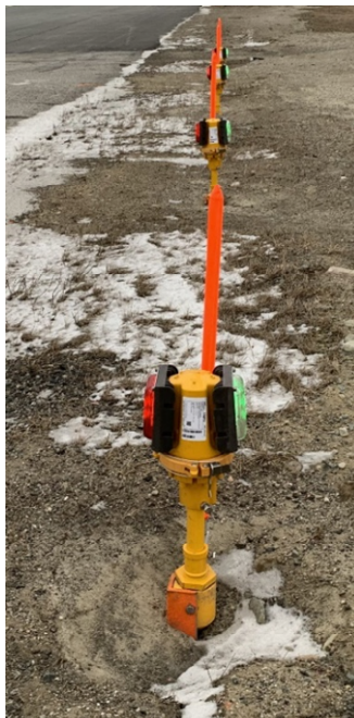
Figure 27- Runways End and Threshold Lights on Runway 04
