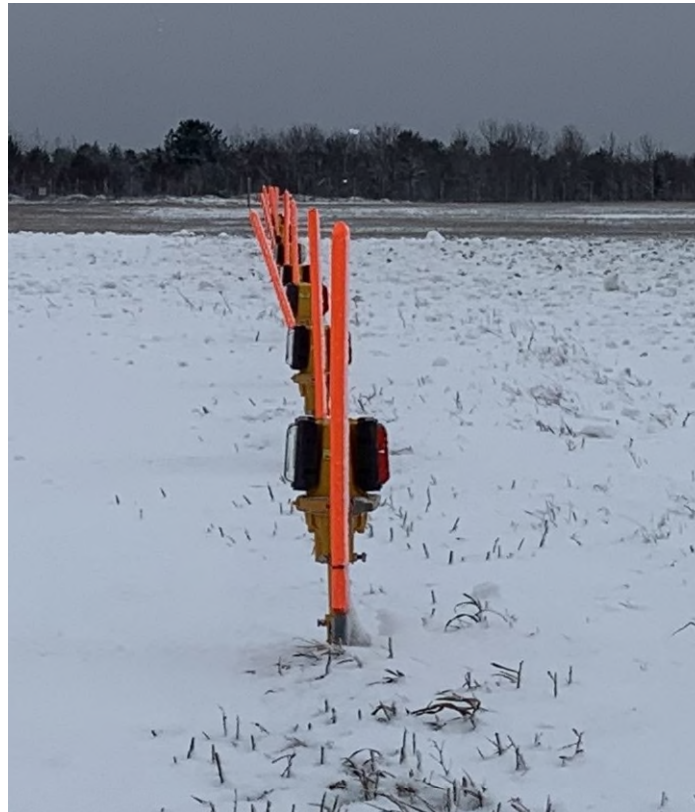
Figure 30 - Runway End and Threshold Lights on Runway 22
