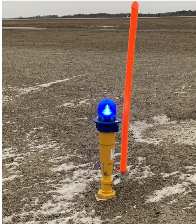
Figure 35 - Taxiway Edge Light Alpha and Bravo
